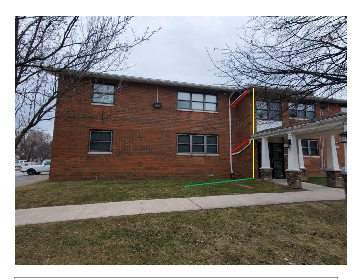
Route new downspouts as indicated by the yellow lines. Run underground feed 15-feet minimum to pop up discharge as indicated by green line. Eliminate connecting downspouts indicated by the red lines. This layout is to apply to all canopied entrances in buildings 4-7 (16 total).
